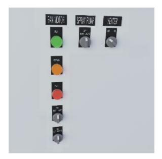
Figure 30 – Typical Control Panel Front Operators
